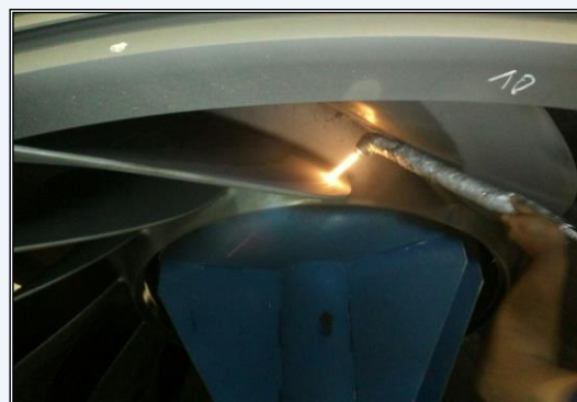
Application of cavitation coating. Chile
