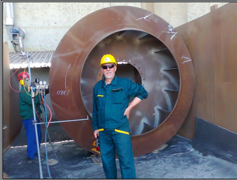
Protect welds seams of smoke extraction turbine from sulfide-oxide corrosion. Coating is NiCrBSi. Bulgaria.
